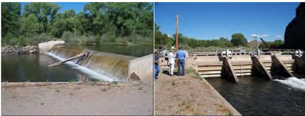
Figure 2-8. Diversion Dam (left) and Head Gates (right) to Rio Grande Canal.
