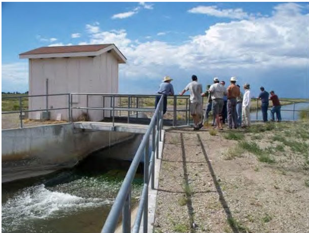
Figure 2-2. Flume at the end of the Closed Basin Project's Main Canal
