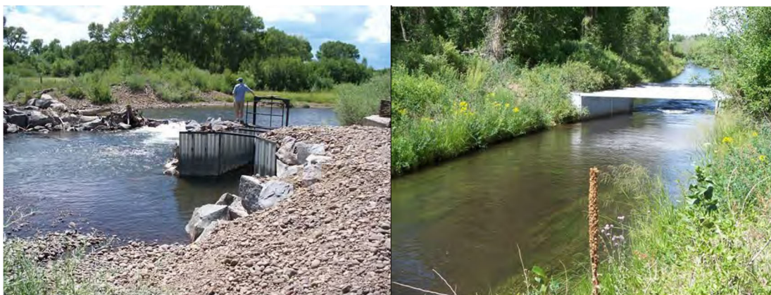
Figure 2-9. Diversion for Romero Ditch (left), and Parshall Flume in Romero Ditch (right).
