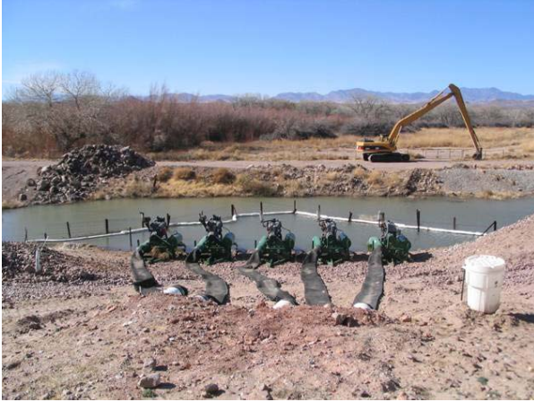
Figure 2.7. Low Flow Conveyance Channel Pumps
